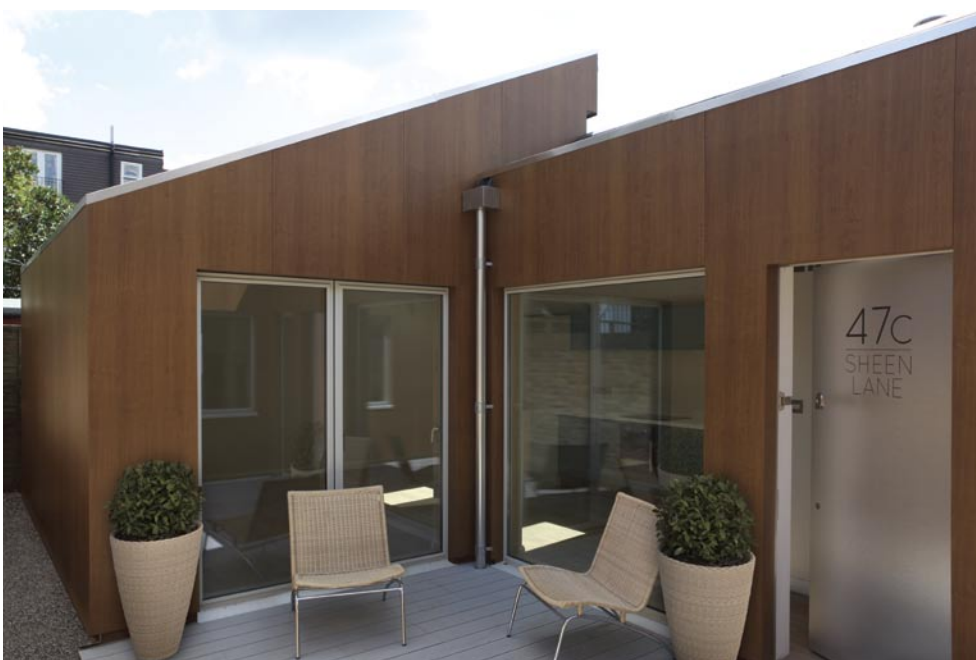
Super-light timber building with no poured slab, southwest London, by Facit Homes
