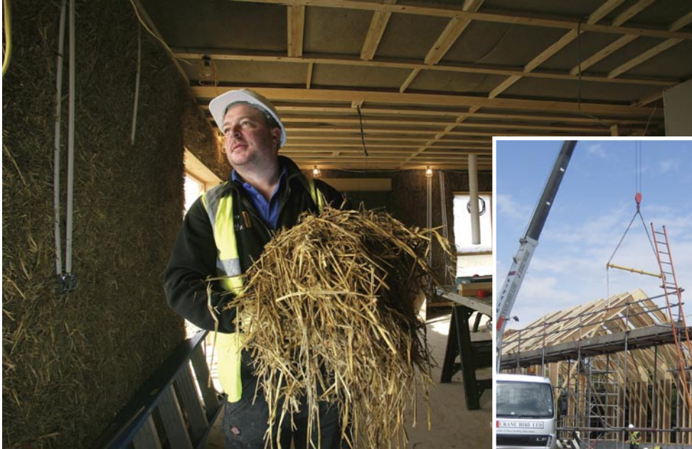
Straw and timber lock up carbon - but should this be subtracted from the other impacts?
